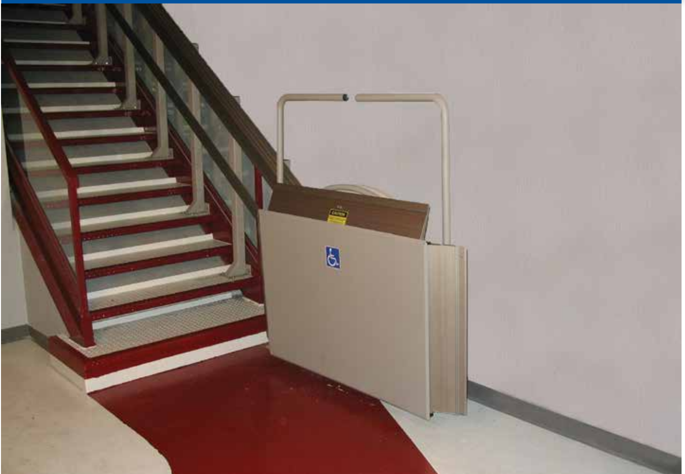
Inclined platform lift for straight stairways
