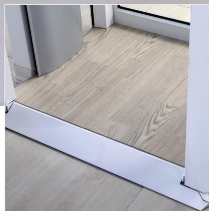
Sloped threshold and attractive non-skid flooring
