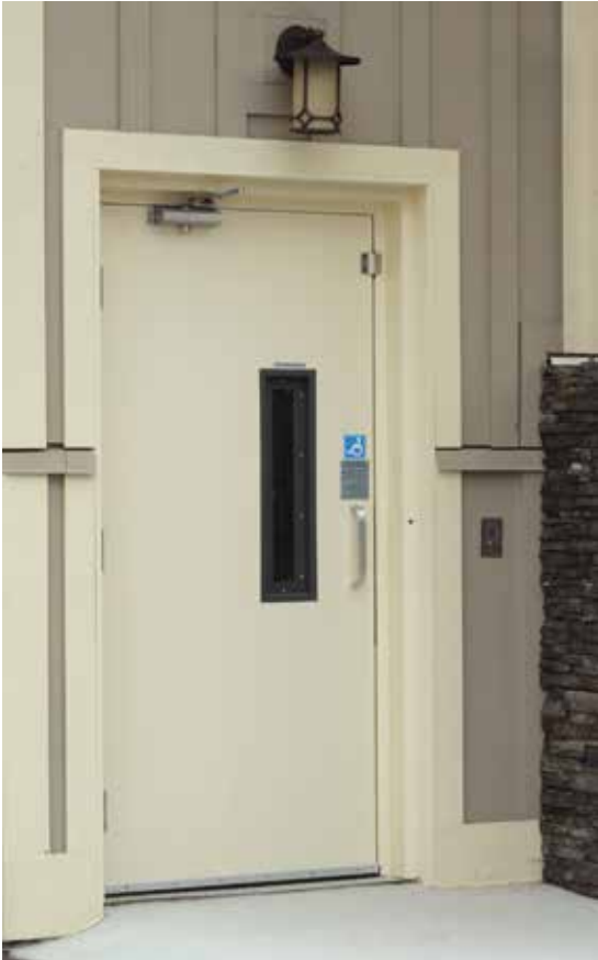
Vertical platform lift with a full height cab
