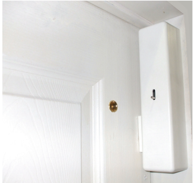
Swinging Door Interlock Shown for Standard and Upgrade Door Packages
