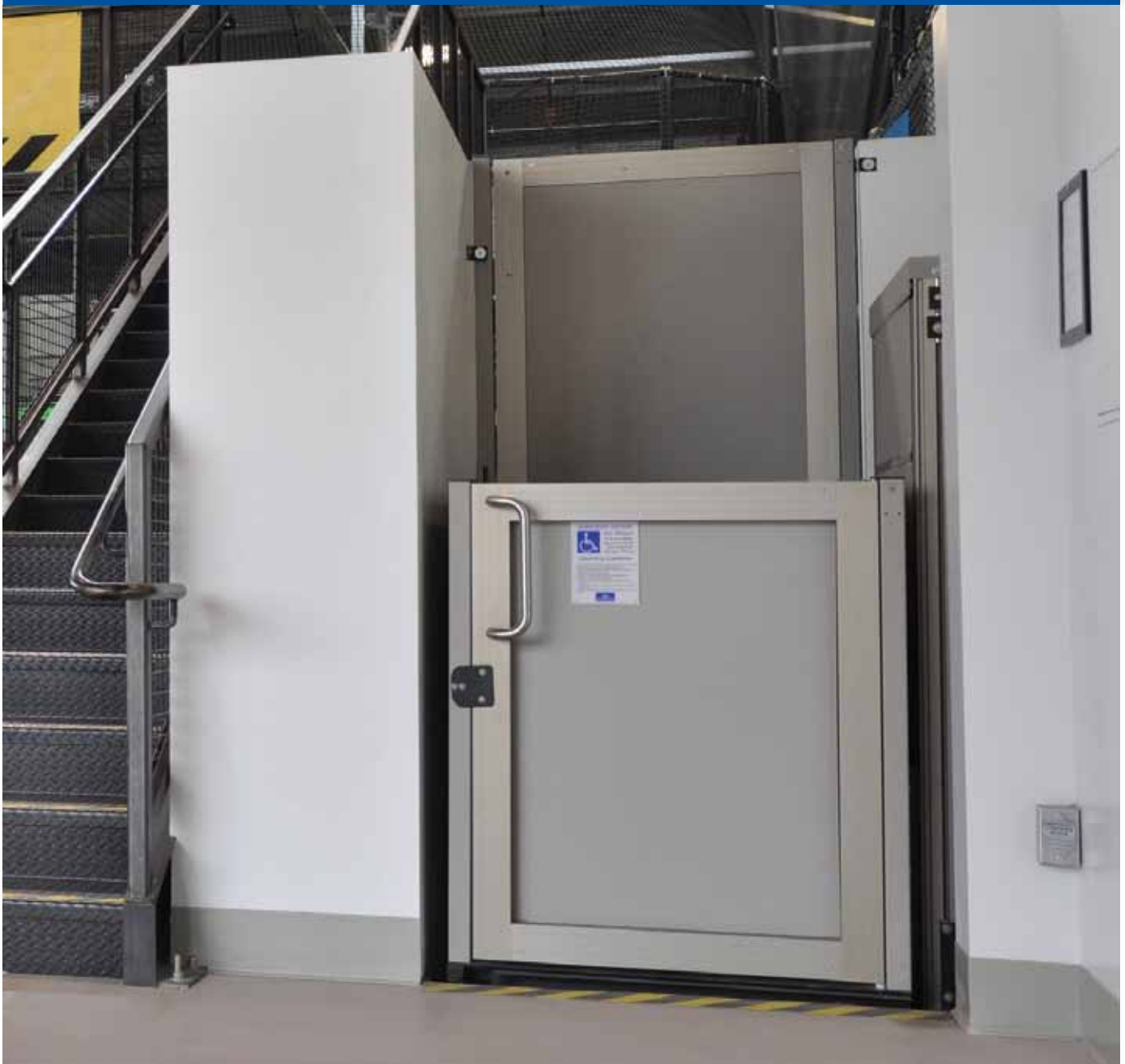
Unenclosed Platform Lift for lifting heights up to 5 feet
