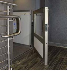
The Garaventa Genesis is a vertical platform lift which provides access into or within commercial or residential buildings. It travels inside a complete, self-contained enclosure, as shown, or can be located in a shaftway constructed by others. Our unique, anodized aluminum design is strong, durable and attractive.
